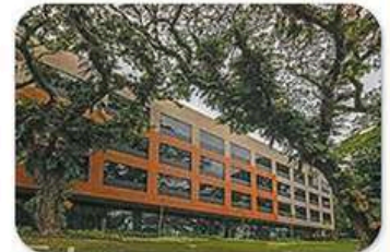
Filinvest Mimosa Leisure Estate Bldg. 4 Longridge Construction Inc.
