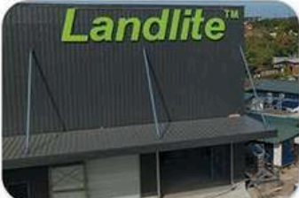
Landlite™ Landlite Headquarters and Warehouse Complex Azienda Fiorento Realty Inc.
