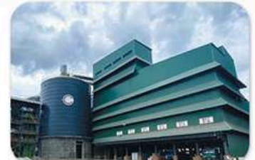
SMC Davao Power Plant San Miguel Consolidated Power Corp.
