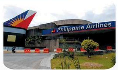
PAL Multi Purpose Bldg. Phil. Electrix Construction Corp.
