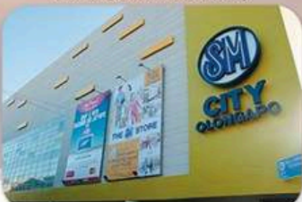
SM City Olongapo / SM Savemore Apalit SM Megamall Carpark Building C SM Prime Holdings Inc. / First Asia Realty Devt. Corp.
