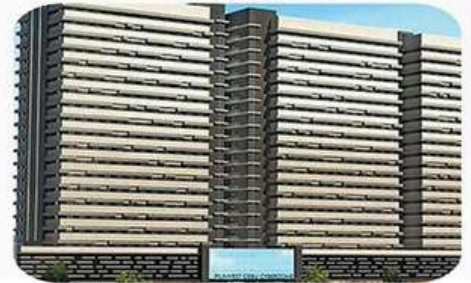
Cebu Cyberzone Mixed Use Tower 3 Integrated Electrical Control Corp.
