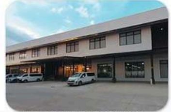
Country Gardens Bataan Avalink Electric & Construction Corp.
