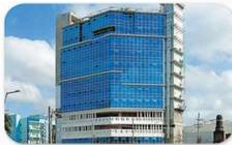
Stronghold Iloilo Logitec Electric & Construction, Inc.
