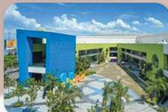
SM City Gen. Santos Main & Carpark Bldg. SM City Davao Expansion Hypervolt Contractor Corp.
