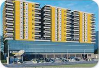
Congbalay 12-Storey Mixed Used Condominium Klaire One Corporation
