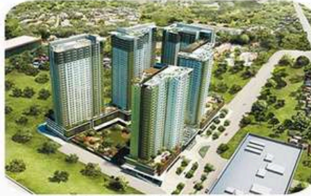
Avida Towers Riala Tower 5 Avida Land Corporation
