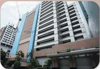
Eastern Telecom Plaza Eastern Communications
