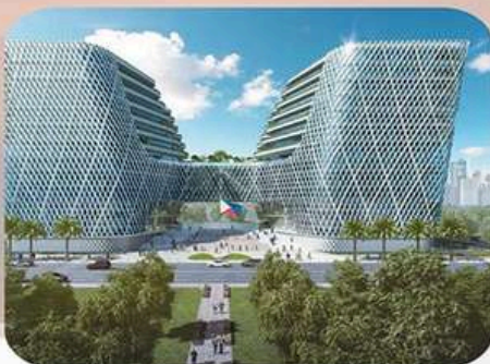
New Senate Building Hilmarc's Construction Corporation
