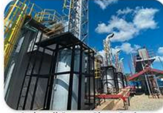
Ardnosil Power Plant Project Ardnosil Const. & General Services Inc.
