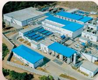
Calawis Water Treatment Plant Makati Development Corporation
