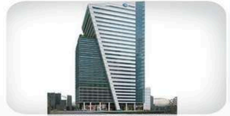
Globe Project- 11 Sites Globe Telecom Inc.
