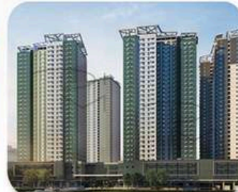
Avida Towers Riala Tower 5 Avida Land Corporation
